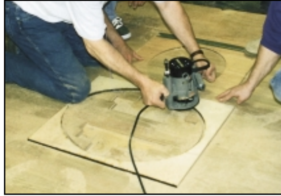
Many companies provide templates with their medallions as a guide to routing the area needed.
