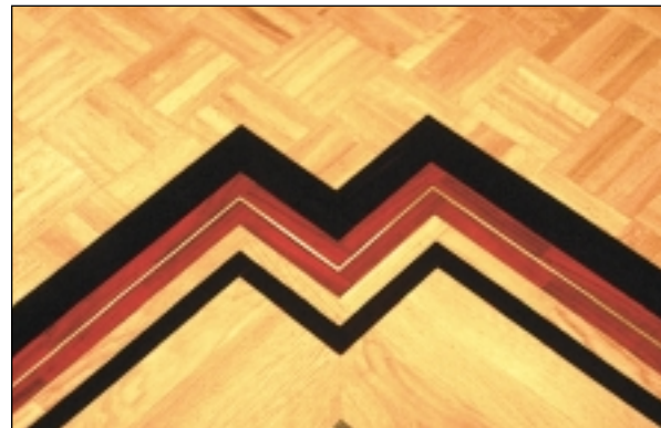
Below, brass is inset in this ebony and padauk border, set in an oak strip and parquet field.
