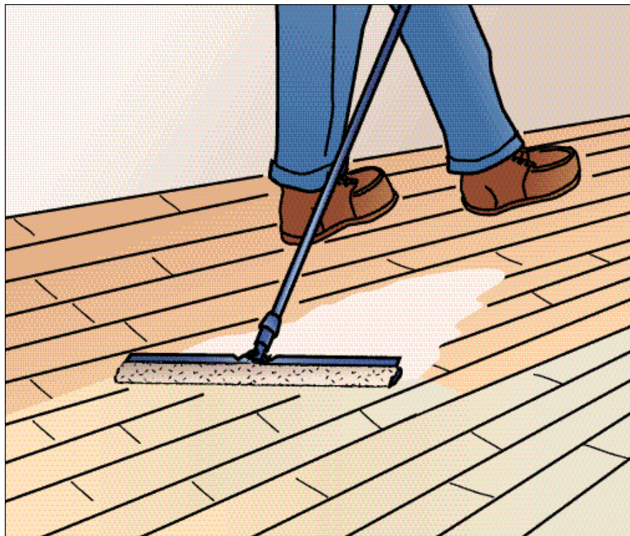
The snowplow method of applying water-based finish
